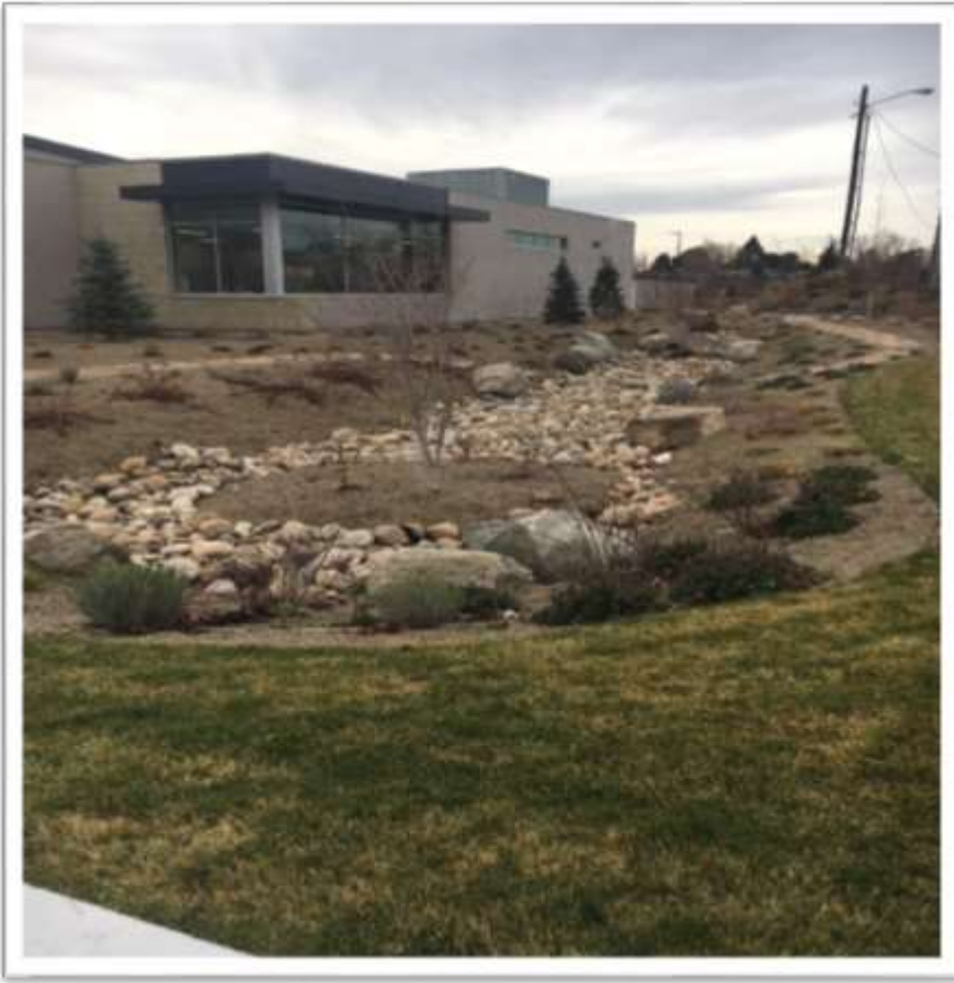
Figure 2: Bown Library Bio-swale Stormwater Facility
