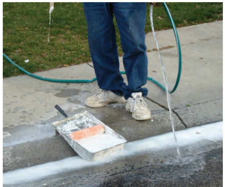
Paint disposal into a gutter, as shown in this picture, is not permitted and is an illicit discharge to the storm drainage system.
