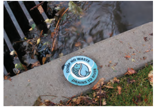
This storm drainage inlet, also known as a catch basin, collects runoff from a street in Downtown Boise.
