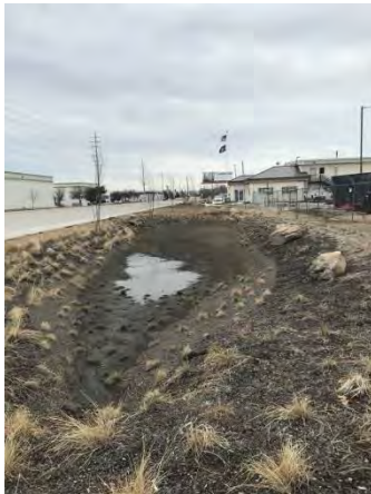
Photos 1-3 from left to right. Drainage area 1 bioretention swale (BRS-1), drainage area 4 bioretention Swale (BRS-4) and Evans Drain outfall (COF1).
