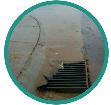
Construction Site Sediment Discharge
