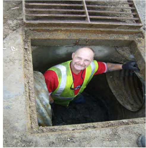
Figure 189. Cleaning a sediment trap.
