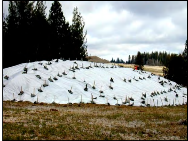
Figure 114. Covered stockpile (ITD 2014).
