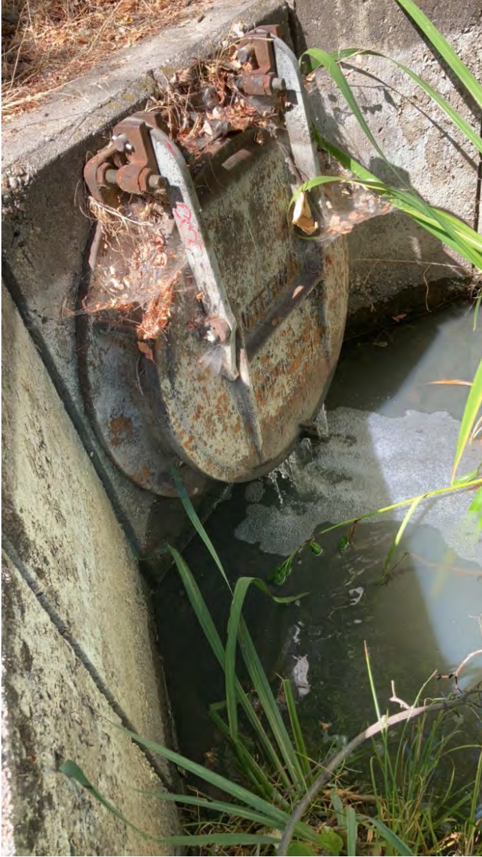
Photo 1: Outfall with closed lid.
