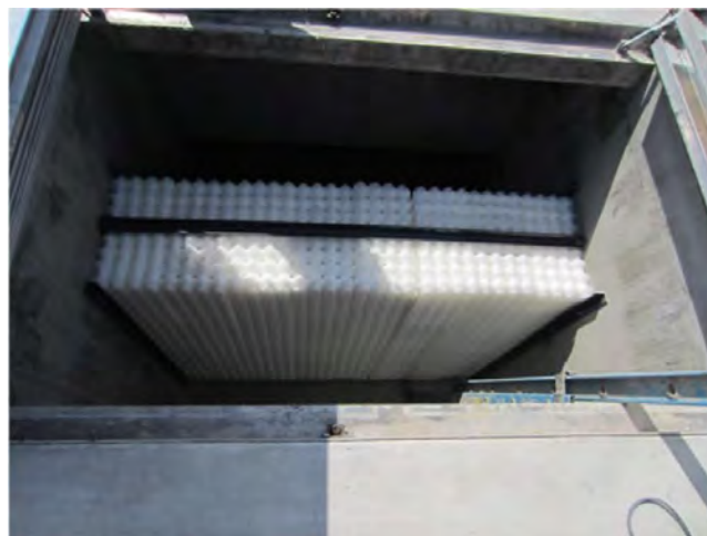
Figure 40. Oil and water separator with coalescing plate separators to remove hydrocarbons ( Mohr Separations Research, Inc. ).
