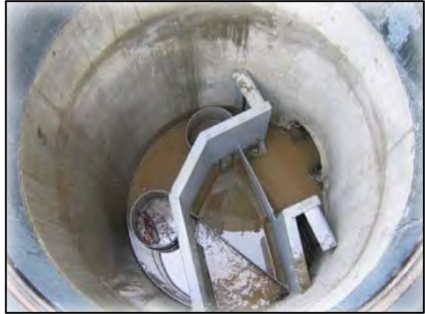
Figure 44. Inside view of Kristar 48-inch dual vortex separator (City of Watsonville, CA).
